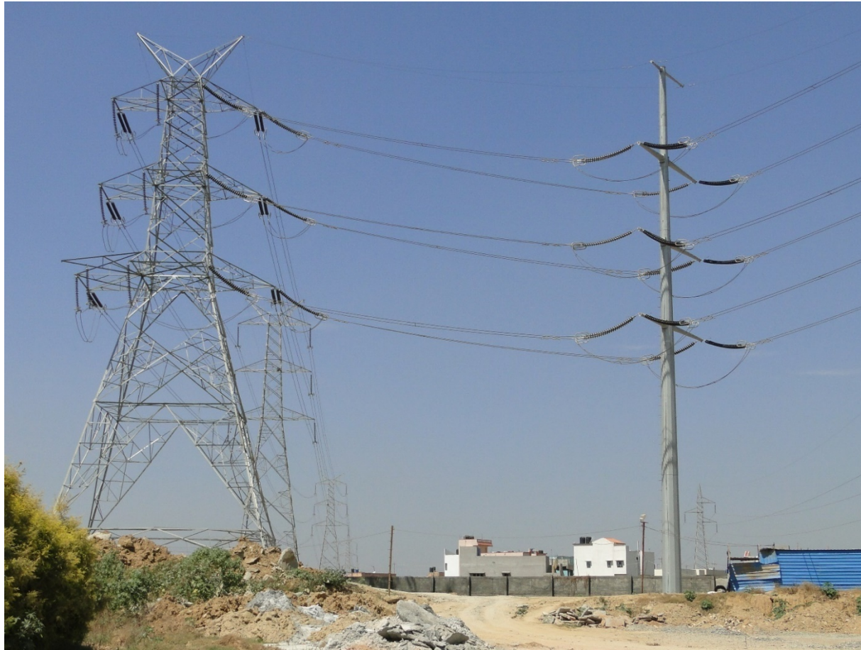
(A) LATTICE AND MONOPOLE STRUCTURE
