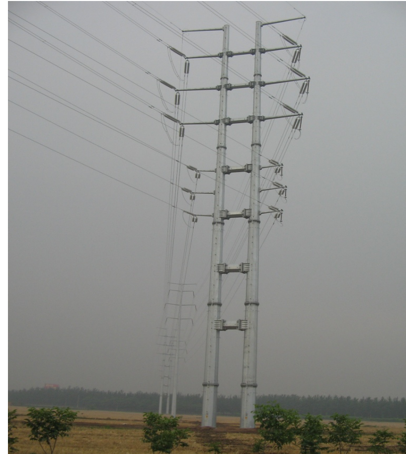
(B) MONOPOLE WITH MULTI CKT & MULTI VOLTAGE
