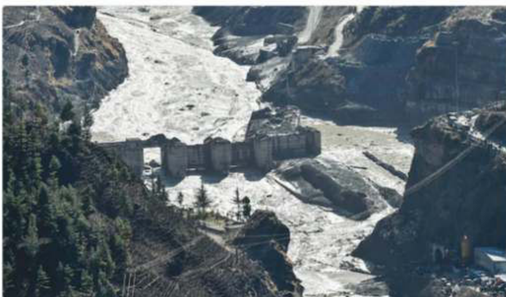
Aerial view of Tapovan barrage two days after a glacier broke off in Joshimath causing a massive flood in the Dhauli Ganga river.
