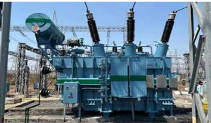
ICT at Pusauli HVDC S/s - Charged after Retro-Filling with Natural Ester Oil
