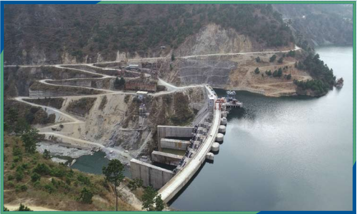
Side view of Bichom Dam, 600 MW Kameng Hydro Power Station, Arunachal Pradesh
