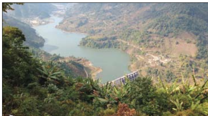
Top view of dam of 405 MW Ranganadi Hydro Power Station
