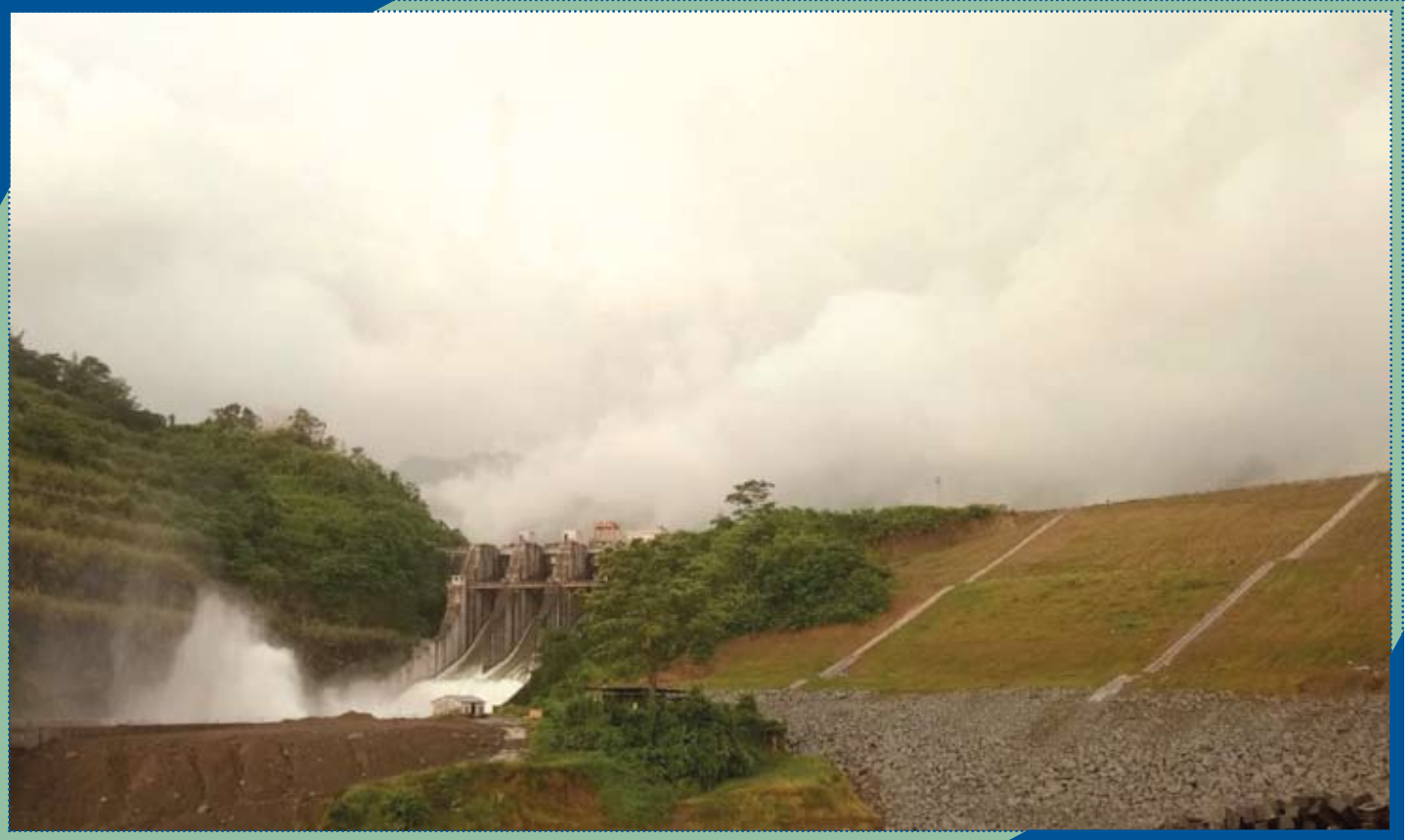
Spillway of 60 MW Tuirial Hydro Power Station, Mizoram
