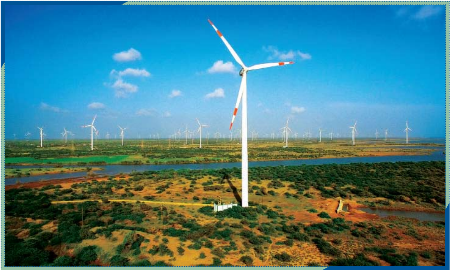
Suzlon wind farm, Bhuj, Gujarat
