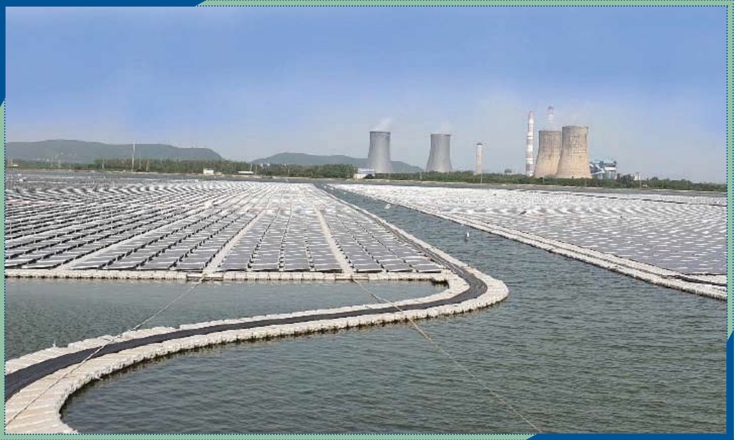
36 MW Floating Solar Project - Visakhapatnam, NTPC
