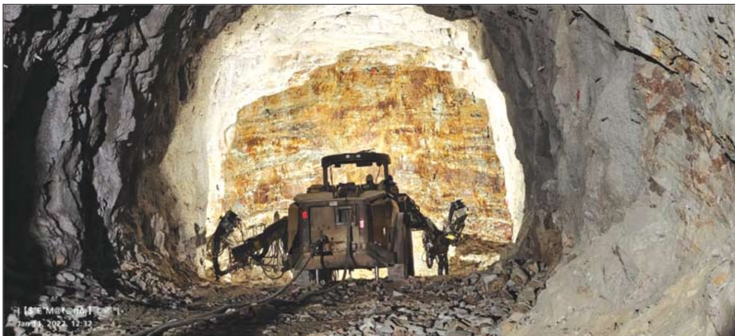
Hrt Excavation – Kiru H.E. Project
