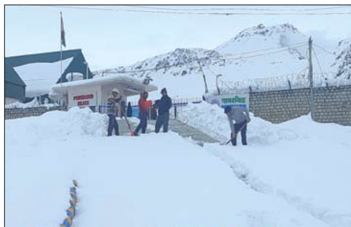
220 kV Drass, Ladakh Substation
