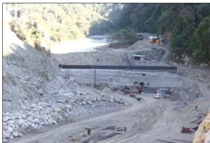
Arun-3 HEP (900 MW) - Coffer Dam Area Construct
