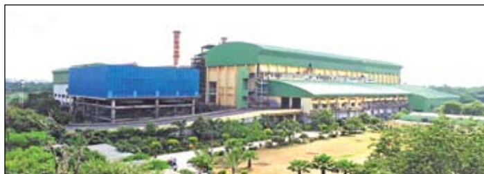
20.9 MW Waste to Energy (WTE) Plant in Bawana Industrial Area, New Delhi funded by PFC
