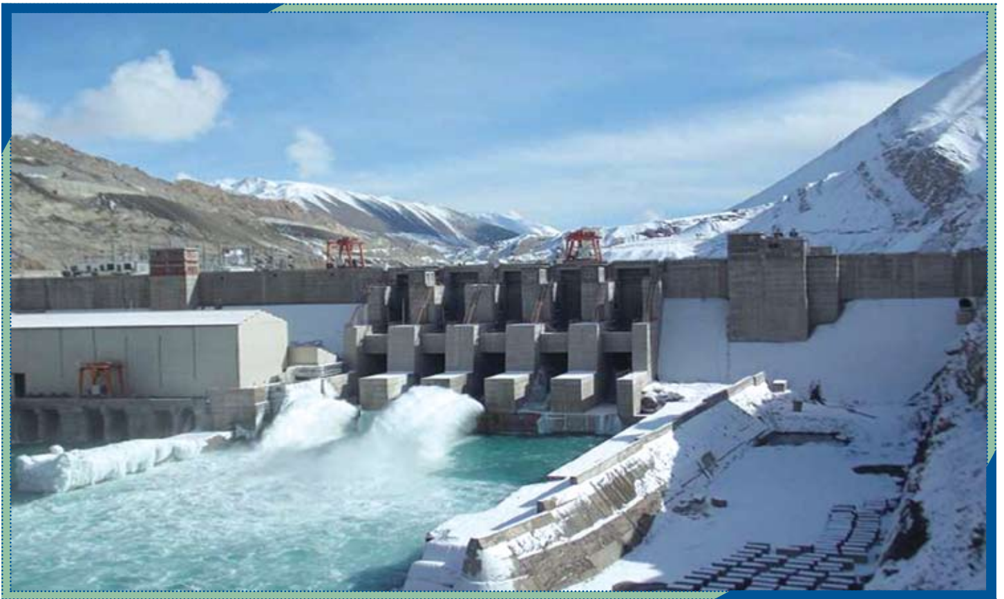
45 MW Nimoo Bazgo Power Station
