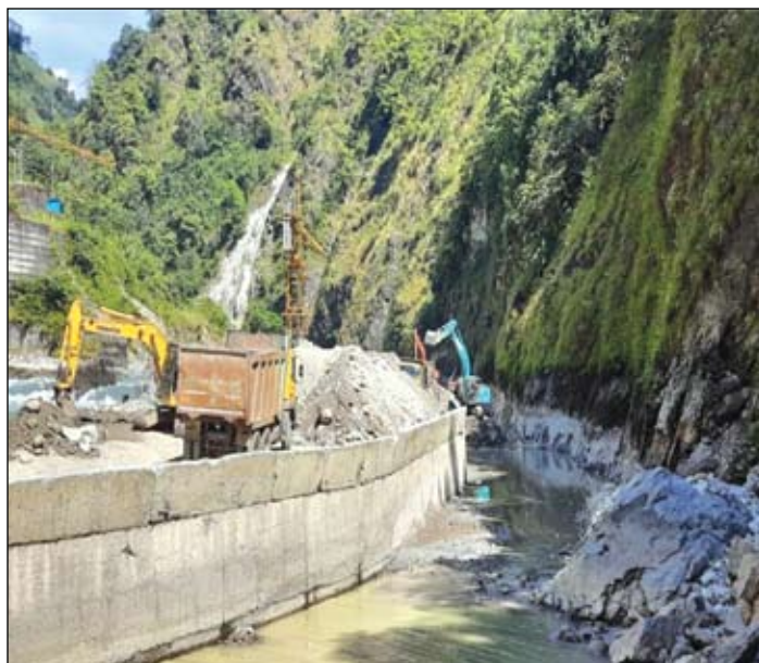
River Diversion - Rangit-IV H.E. Project
