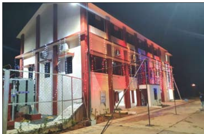
First GIS Substation of Goa (Davorlim-Navelim) virtually inaugurated by Hon'ble PM on GOA Liberation Day, 19 December 2021
