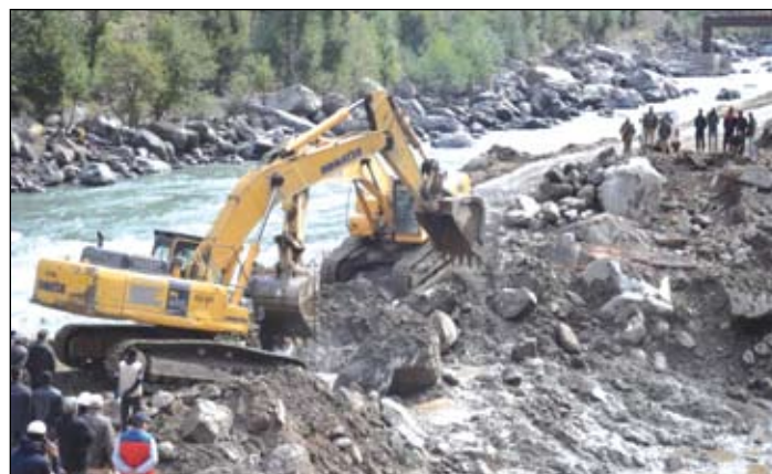
River Diversion - Pakal Dul H.E. Project
