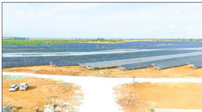
35 MW Babsar Site funded by PFC
