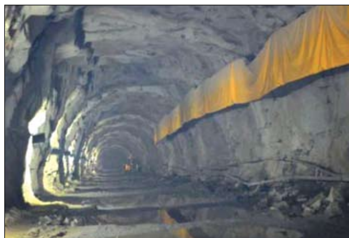
Luhri Stage-1 HEP (210 MW) - Diversion Tunnel Construction
