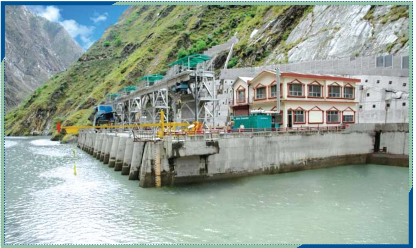
1500 MW Nathpa Jhakri Power Station
