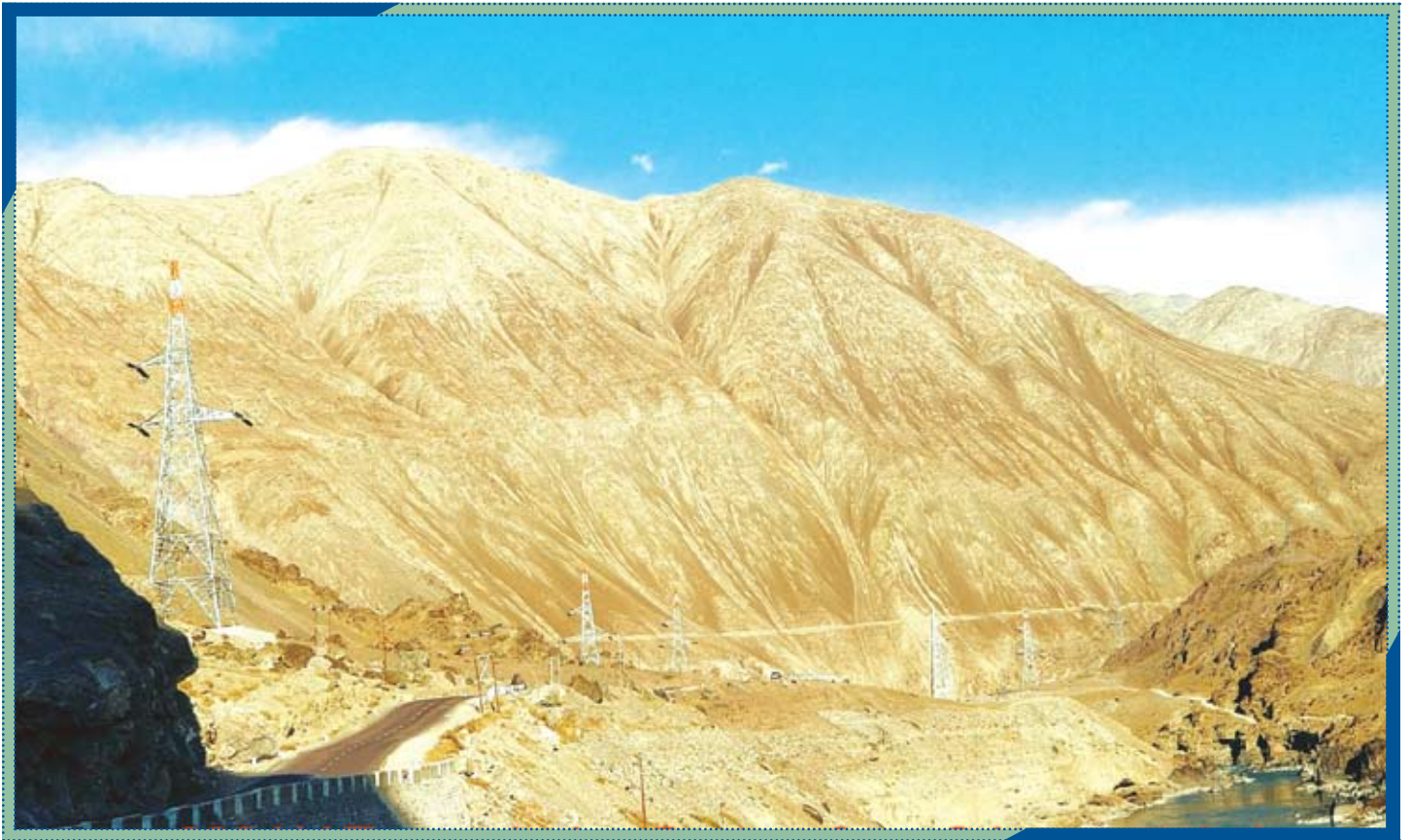
220 kV Transmission system from Srinagar to Leh
